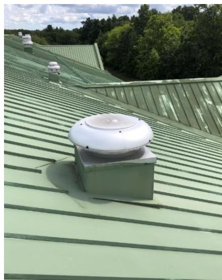
Picture 5: Multiple inspected EFs on the roof
