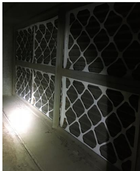
Picture 2: AC1 Dirty MERV 8 Filters
