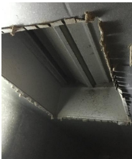
Picture 3: AC1 closed OA damper
