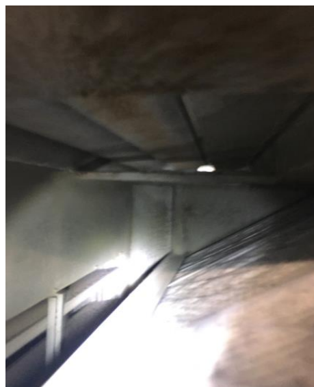
Picture 4: AC2 partially open OA damper
