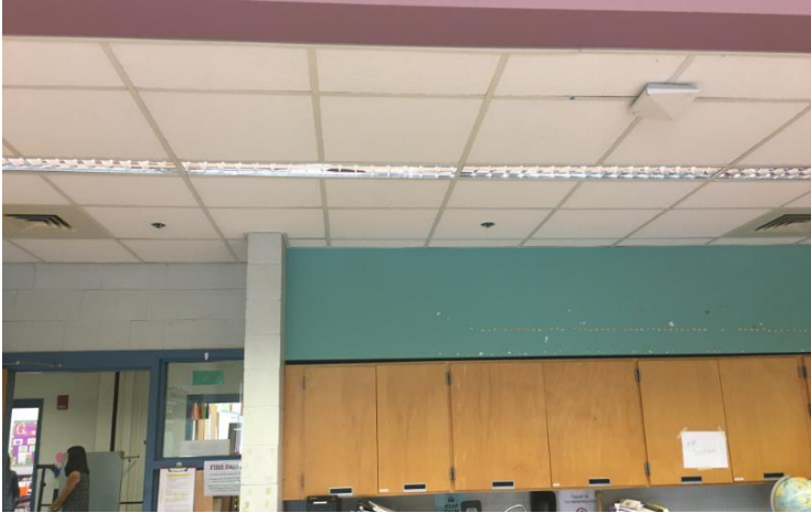
Picture 7: Typical exhaust setup with transfer grill left and exhaust grill right
