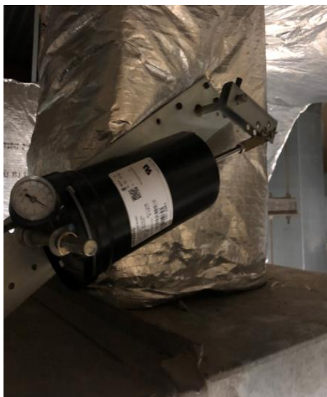
Picture 1: HV1 OA Damper Actuator pressure gauge (15PSI)
