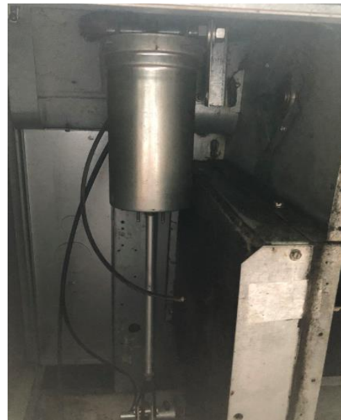
Picture 12: Disconnected OA Damper actuator Rm 221
