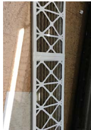
Picture 9: Filter requiring replacement Rm 108
