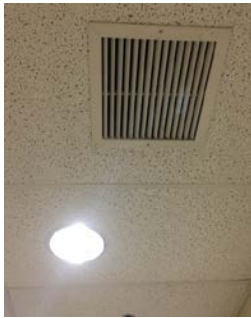
Picture 5: Typical Bathroom Exhaust
